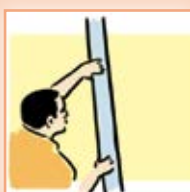
Making walls plumb.
